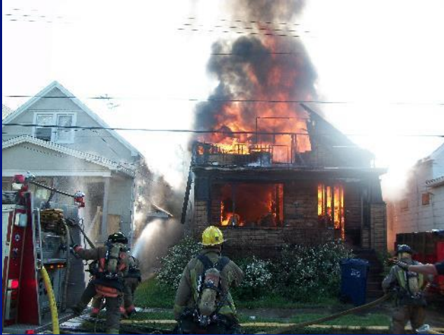
Residential fire (photo by IAFF.org)
