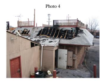
The two additions had wood frame roofs which abutted the original building's façade. The roofs were covered with standard asphalt shingles. See Figure 1 for the floor plan.
