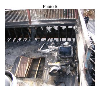
The fire spread from the ventilator to the back side of the building's decorative façade. The fire burned into the void space within the façade, and spread around the entire façade.
